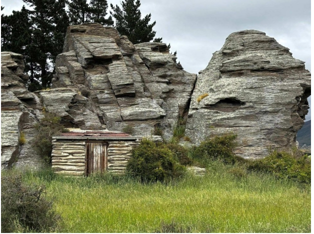
Derelict schist hut (photo by Helen Emerson)
